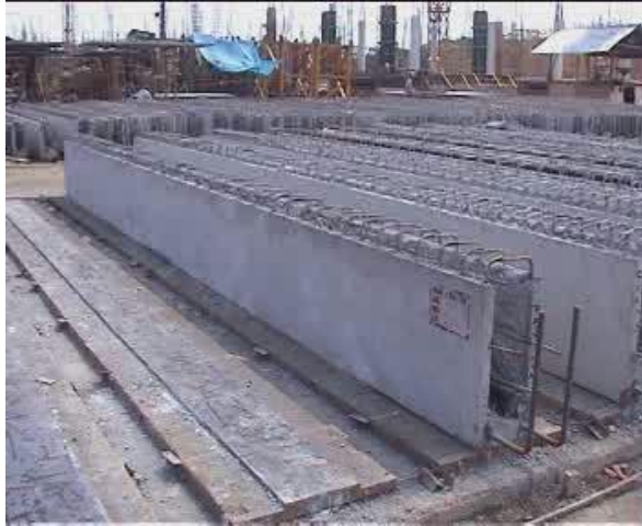
Gambar 2.3 Balok Precast U-Shell Sumber: Juklak PT. PP Persero (2014)
