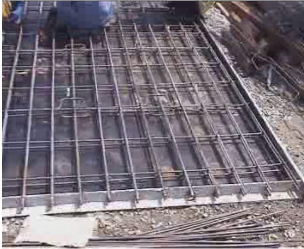
Gambar 2.4 Produksi Half Slab Precast Sumber: Juklak PT. PP Persero (2014)
