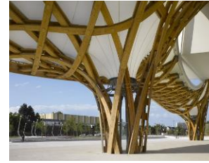
Gambar 15. Penunpu Atap Pompidou Centre Metz Sumber: https://www.centrepompidou-metz.fr
