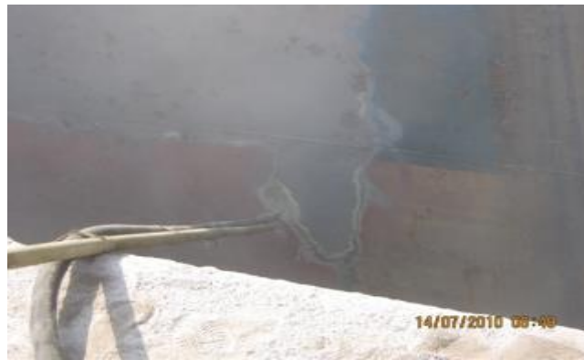
Gambar 2.2.B Proses Blasting
