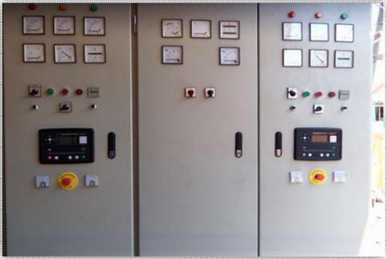
Gambar 2.7 Panel Automatic Transfer System
