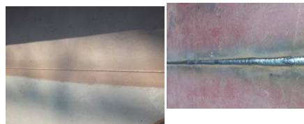
Gambar 10. Finishing Joint Block Metode Stopper Manual.
