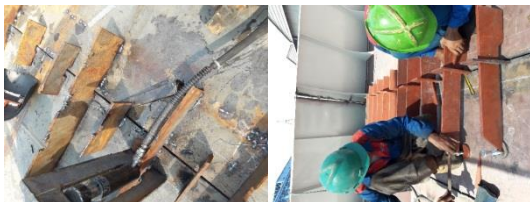
Gambar 8. Fitting Block Metode Stopper Manual.
