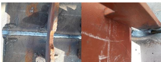
Gambar 9. Welding Joint Block Metode Stopper Manual.
