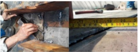
Gambar 7. Adjusting Block Metode Stopper Manual.
