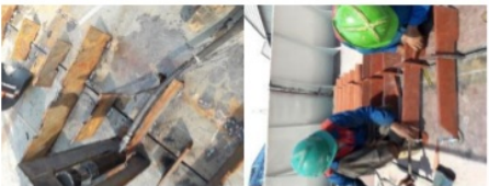
Gambar 8. Fitting Block Metode Stopper Manual.
