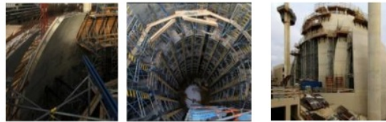
Figure 11. The formwork and reinforced concrete material cast-in-situ [19]
