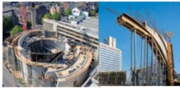
Figure 10. Several concrete shell segments gradually growing together and meet to form a cantilever [18]
