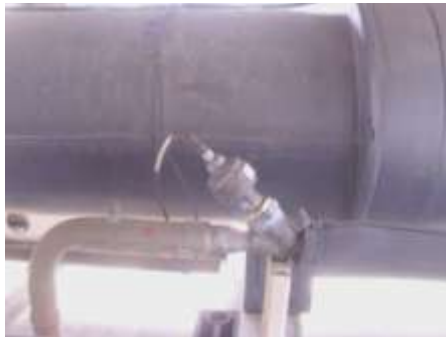
Gambar 4.3. Expansion Valve
