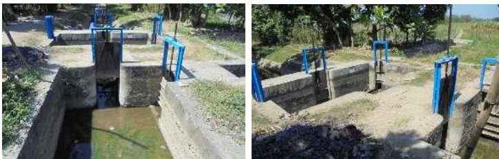
Gambar 4. 2 Bangunan Bagi Sadap (B.LK.2)
