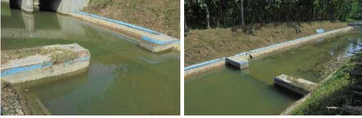
Gambar 4. 4 Bangunan Ukur (B.KN.1c) Sumber : Hasil Penelusuran Jaringan Irigasi, 2020
