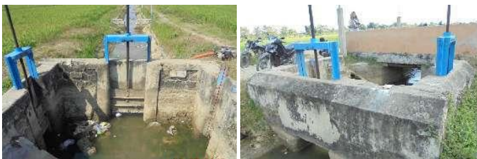
Gambar 4. 3 Bangunan Sadap (B.KM.1)
