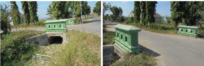
Gambar 4. 9 Bangunan Gorong - gorong (B.BN.2g) Sumber : Hasil Penelusuran Jaringan Irigasi, 2020
