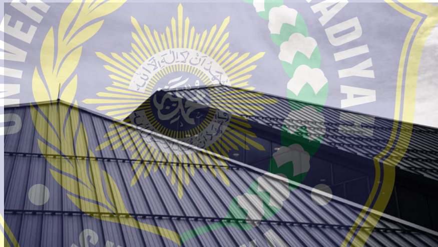
Gambar 5. 7 Material atap : multiroof galvalume steel (Sumber : https://www.rumah.com/panduan-properti/jenis-atap-rumah-multiroof-63093 , 2023)
