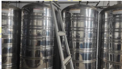
Gambar 4. 8 Tandon Stainless (Tandon Jadi) (Sumber: PT. UMSurya Bina Bangsa)
