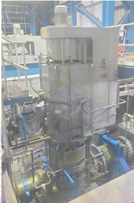
Gambar 2. 1. Condensate Extraction Pump (CEP)
