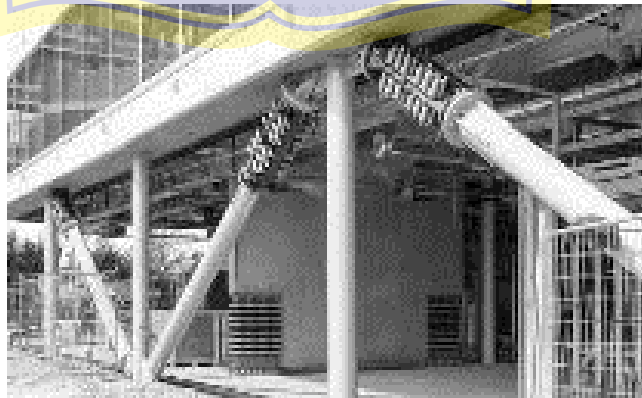
Gambar 2.19 Seismic bracing . Sumber: Tectonus (2022)
