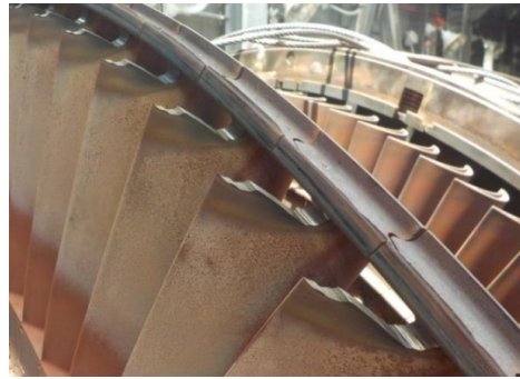
Figure 11. Turbine Stage 2 Bucket Damage before MI CTG 101
