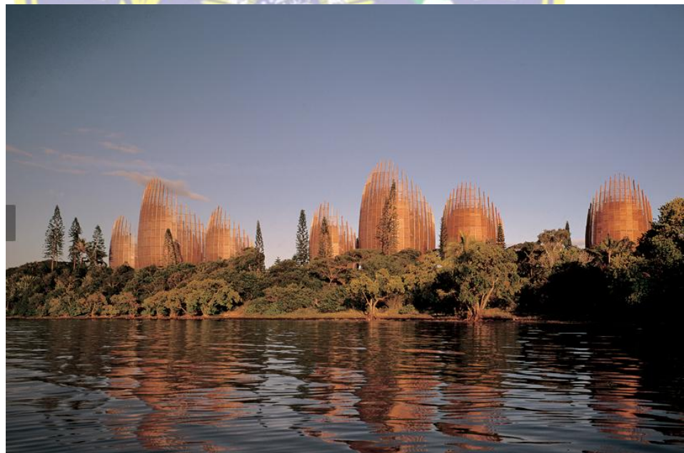
Gambar 2. 14 Fasad Tjibaou Cultural Center (Sumber: https://id.pinterest.com/pin/28991991340734475/ 2026)
