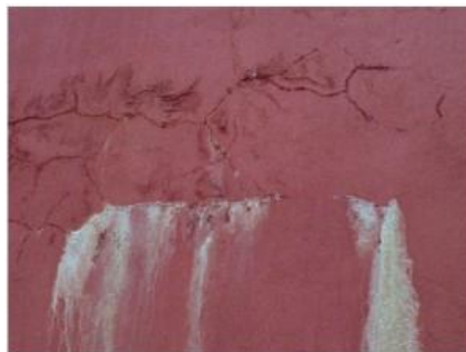
Gambar 2.13 Safonification
