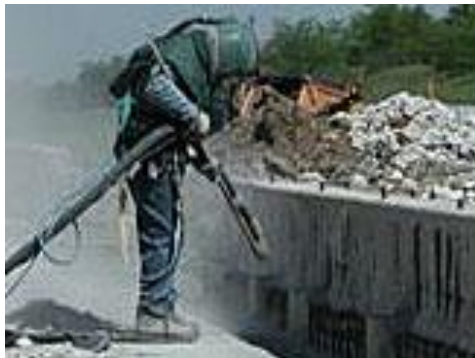
Gambar 2.1 Wet abrasive blast cleaning
